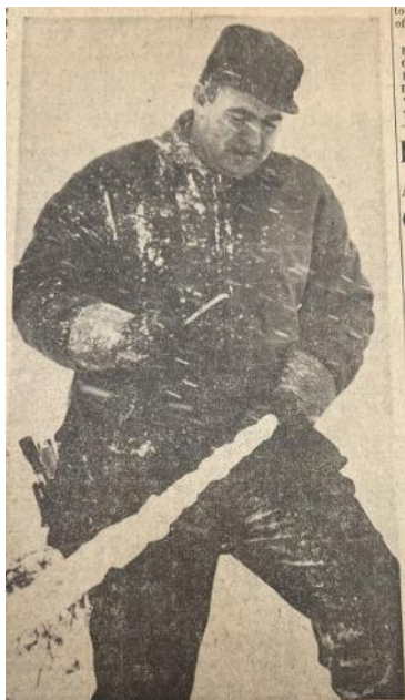
JERRY STORK had his work cut out for him Saturday by Mother Nature as icy snow felled telephone lines in many sections of the county. Freezing temperatures made chipping away the ice a long, cold and slow process. The above photo was taken Saturday afternoon in the McKean area and similar scenes were repeated in many places.
